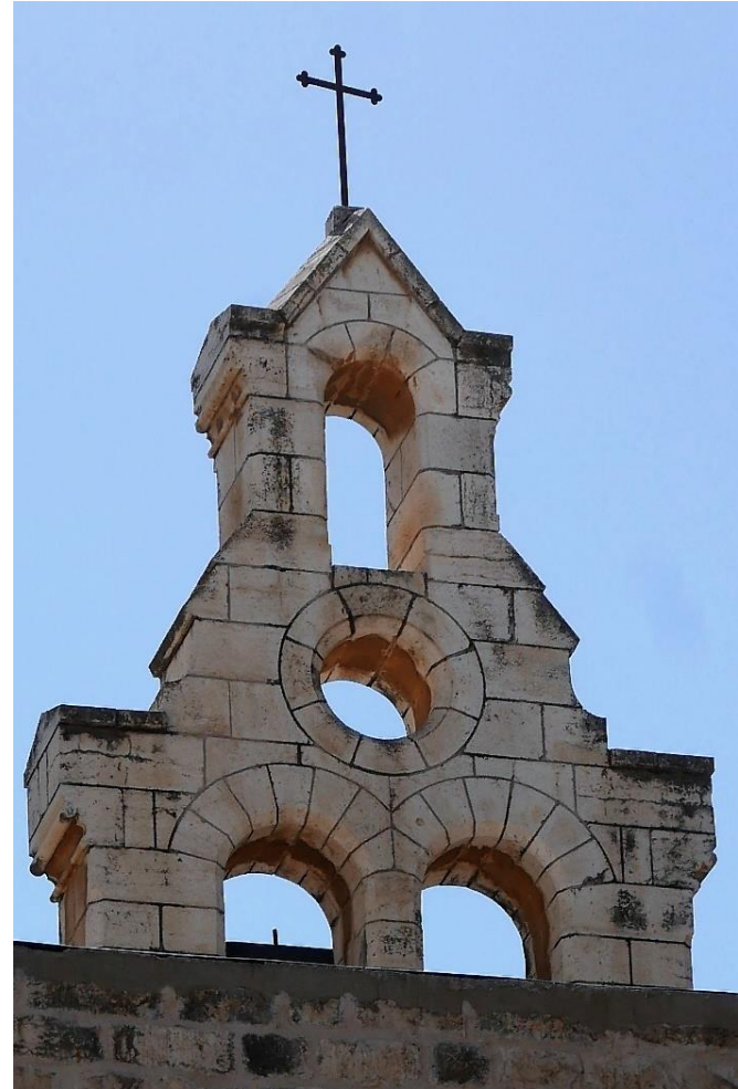
Bell tower Located on the convent's roof
