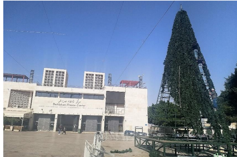
Christmas Tree being erected in mid-November
