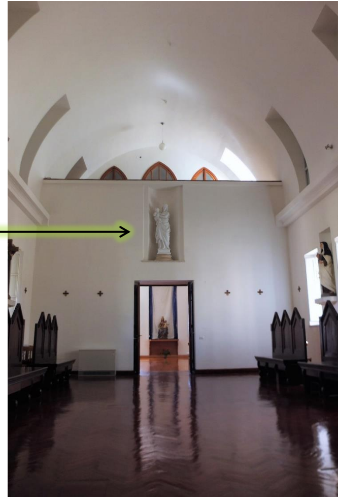
Barrel vault ceiling
