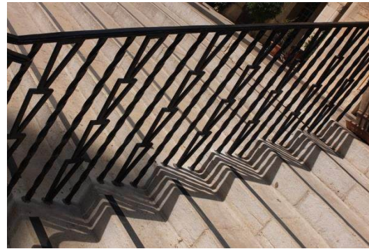
Handrail Entrance plaza
