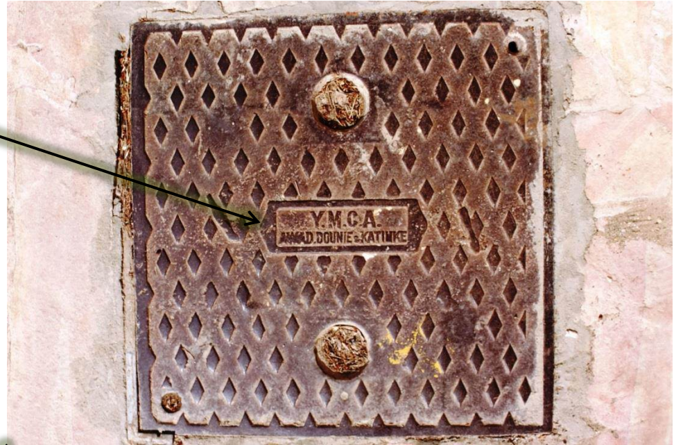
Manhole covers were tailor-made for YMCA and bear the contractor's name
