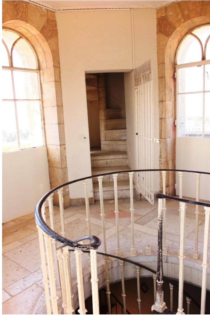
Entrance from Observation floor
