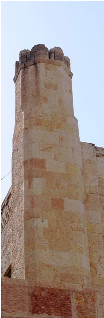
Chimney Western façade
