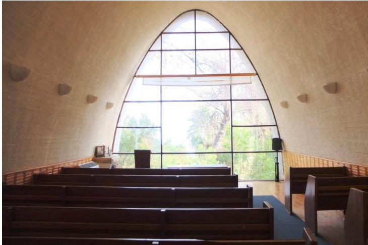
Eastern wall – no apse
