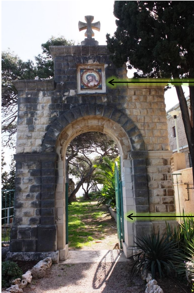
Entrance - Eastward view
