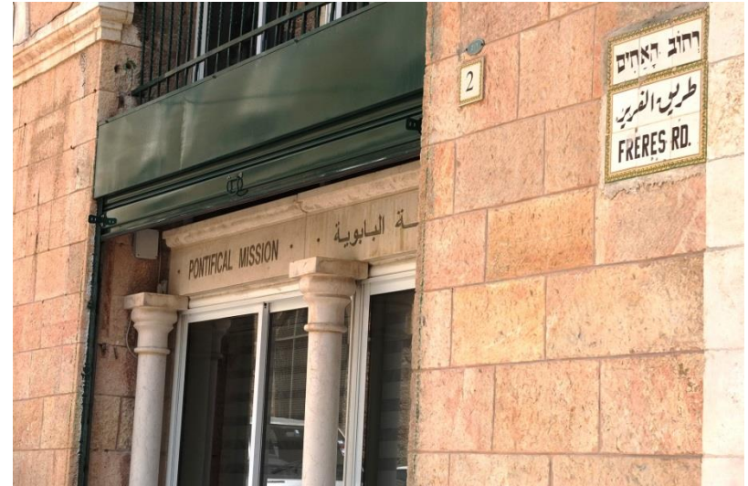
Office at 2 Freres Road
